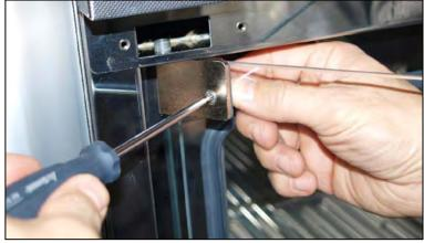
13. Screw the locking pieces tight on the upper and lower right side of the appliance.
